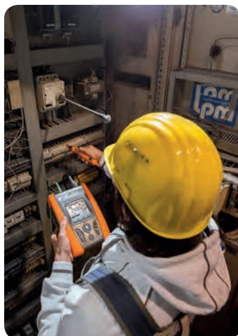
Start/stop measuring with remote lead
